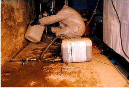
Preparing pump for injection
