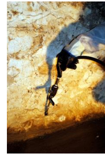
Injection wand attached to packer
