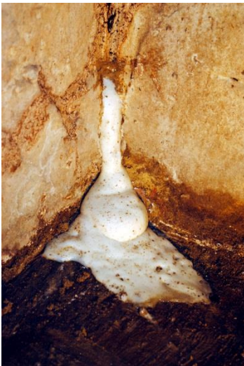
As HyperFlex reacts and fills the void, foam is visible at the injection site.
