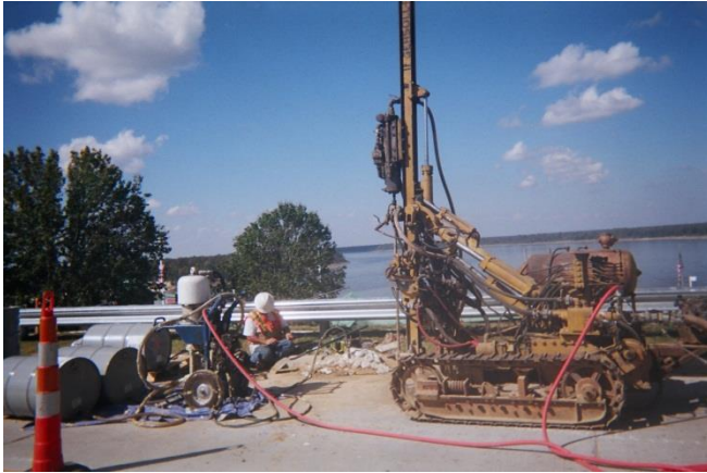
This is our air track machine used to drill bore holes.
