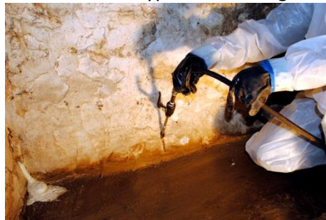
Injection in process. Note how HyperFlex has migrated into the corner
