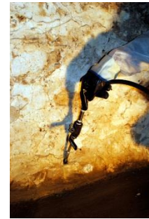
Injection in process. Note how HyperFlex has migrated into the corner
