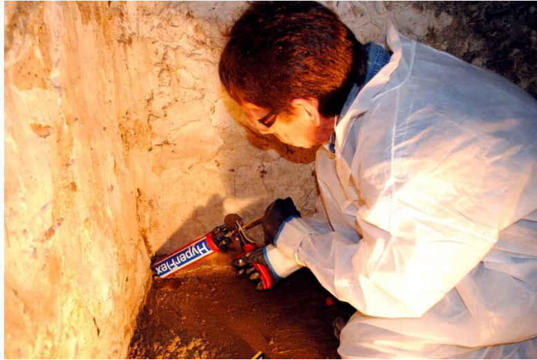
In this photograph, HyperFlex is being used to fill a void found on the other side of this very old farmhouse wall.
