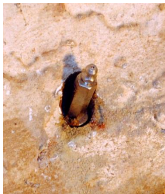
A properly installed 5/8” packer.
