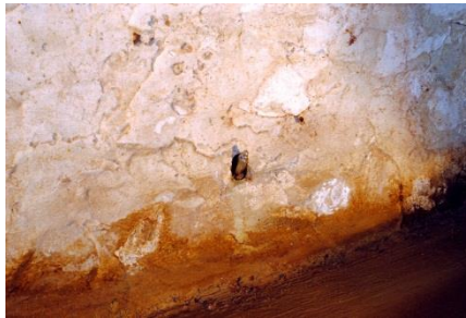
Injection in process. Note how HyperFlex has migrated into the corner
