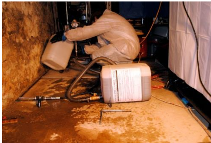
Injection in process. Note how HyperFlex has migrated into the corner
