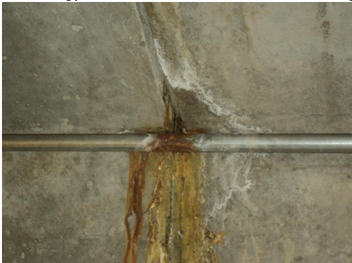
This is an example of the corrosion and rusting of the electrical conduit in the tunnel prior to injection.
