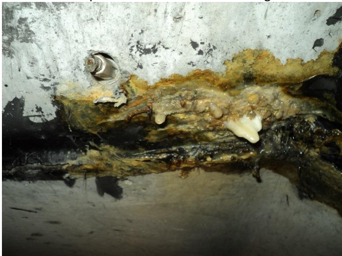
This is an example of the corrosion and rusting of the electrical conduit in the tunnel prior to injection.
